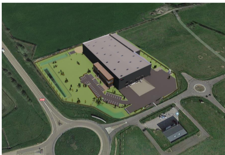
Endupack will occupy nearly two hectares in the Maison rouge area, along the departmental road 438.
